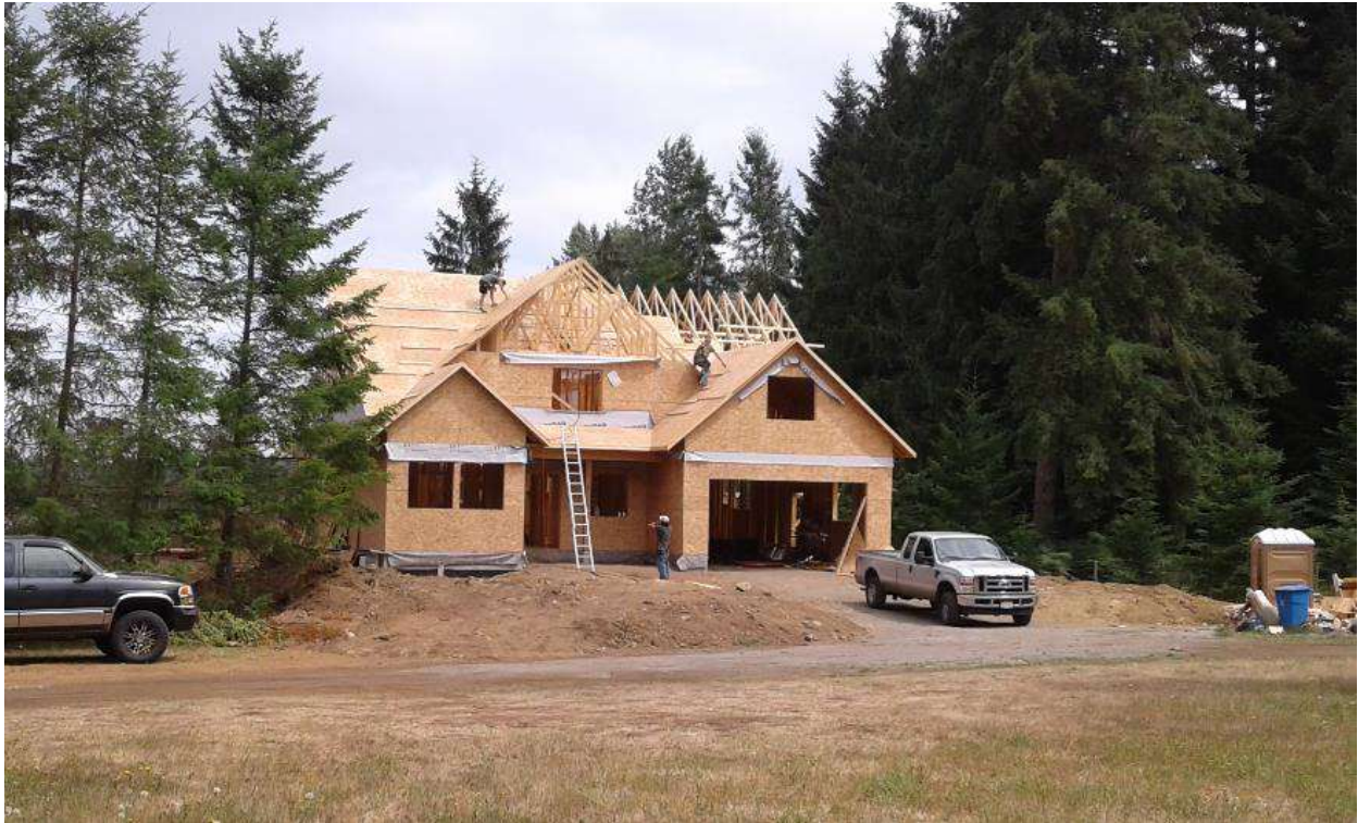
Figure 3: The House at 3719 Cameron Road under Construction (July 5, 2019)
